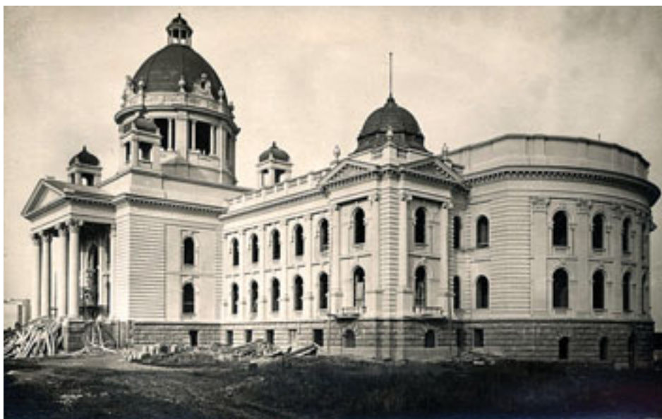
Assembly building upon completion of construction works. The edifice was completed and consecrated on 18 October 1936.
