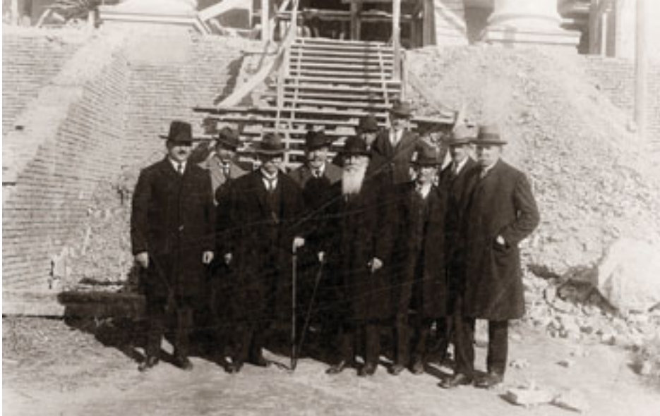
Nikola Pašić with his associates in front of the Assembly building under construction
