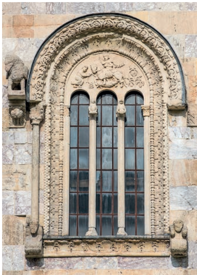
FIG. 159. DEČANI MONASTERY, CHURCH OF CHRIST PANTOKRATOR, WESTERN FAÇADE, THREE-LIGHT WINDOW
