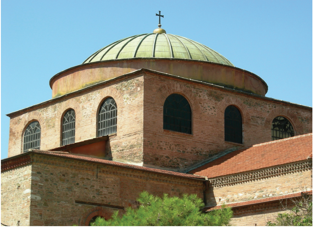
Figure 14. The prismatic middle zone of the tetrapylon core protruding through the roof of the church and supporting a shallow round drum of the dome; Hagia Sophia, Thessaloniki, late 6th or early 7th century
