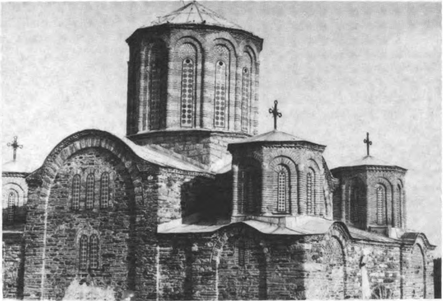
Matejič, upper part of the church, northwest view
