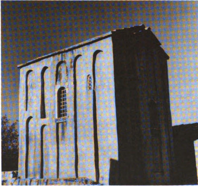
St. Michael near Ston, northeast view
